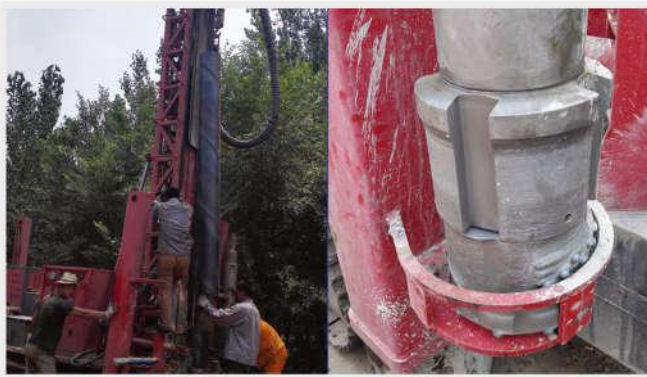
Water Well Drilling
